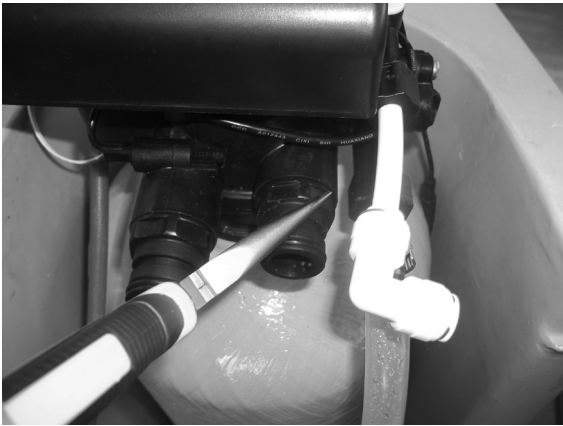
Fig. H - Long Adapter installed
