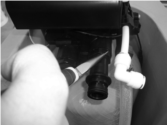
Fig. H - Long Adapter installed
